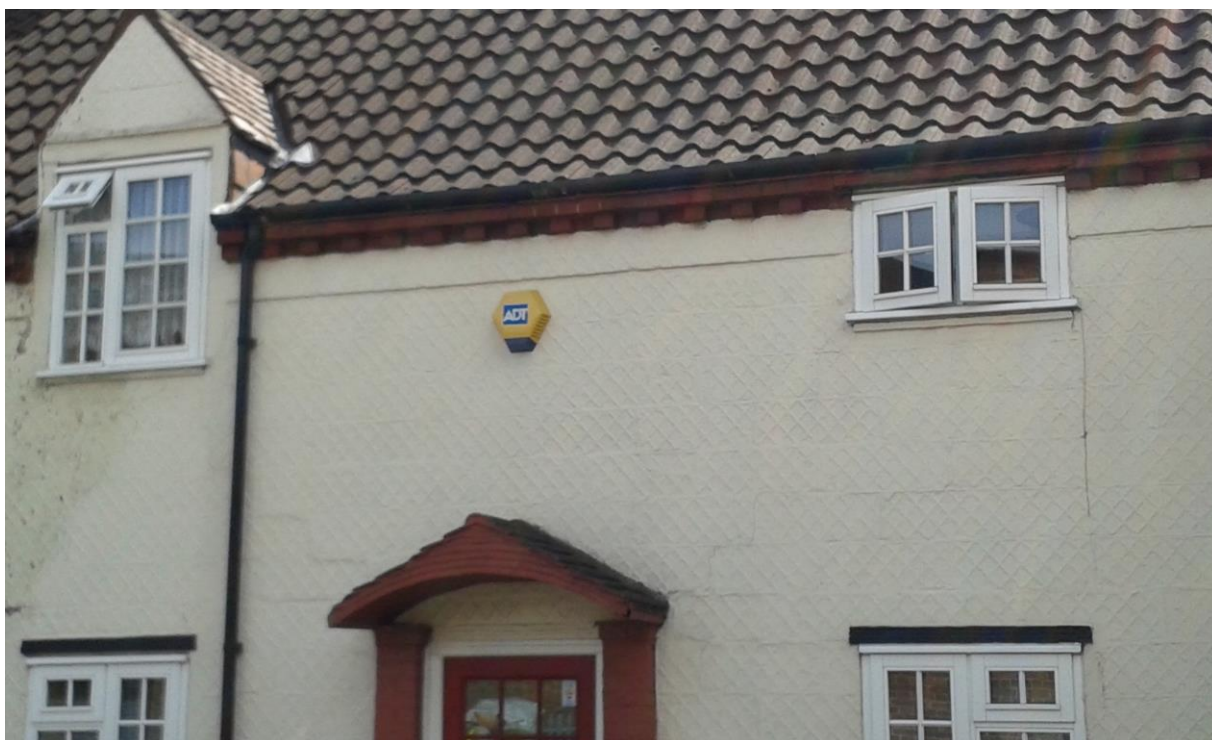
Original patterned stucco and pantiled roofs, Nos. 1-5 (odd) Norbroke Street.
