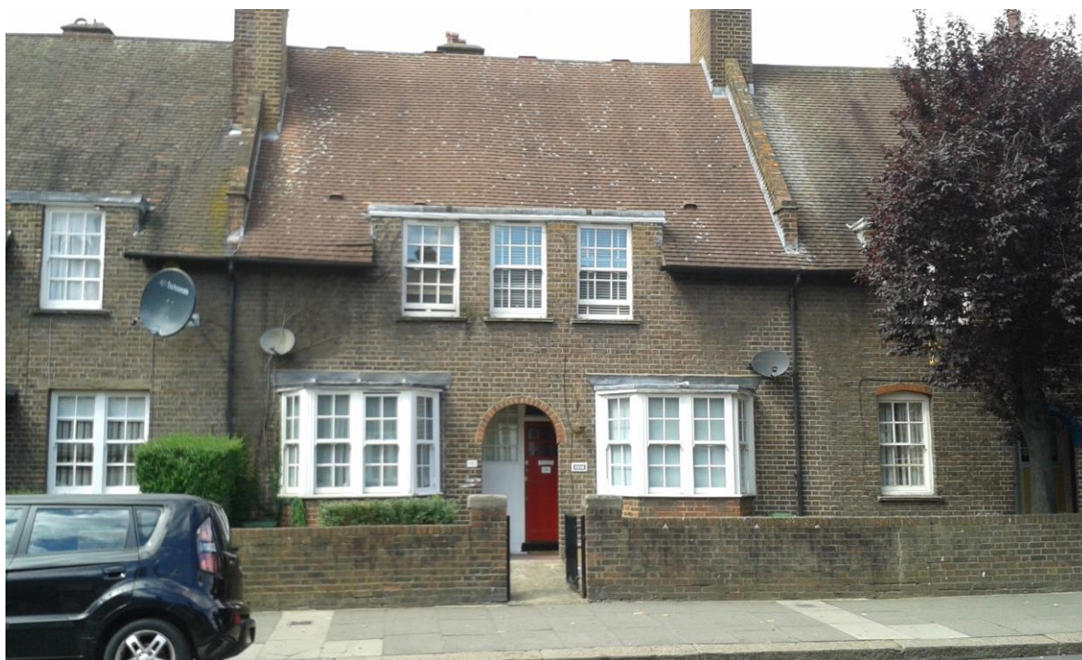
Nos. 33-39 (odd) Erconwald Street, canted ground floor window bays and first floor windows projecting through the eaves.
