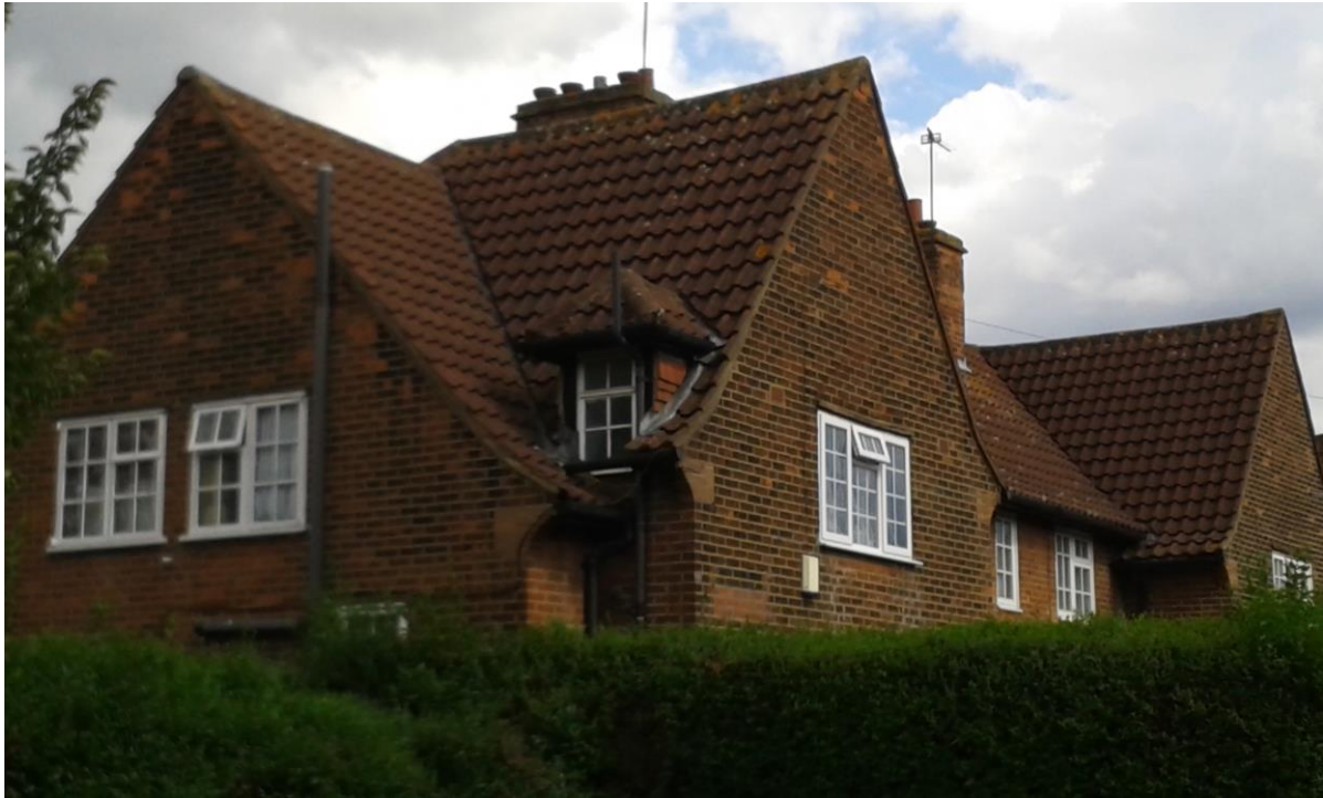
Small dormer projecting from behind the pantiled roof gable. Wallflower Street.
