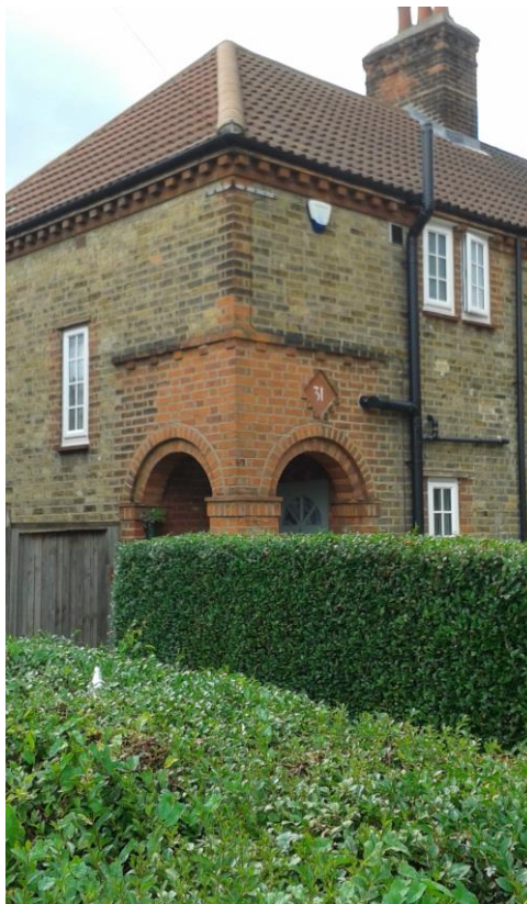
Porch detail: Corner porch with double brick arch and brick dentil string course above. Clematis Street.
