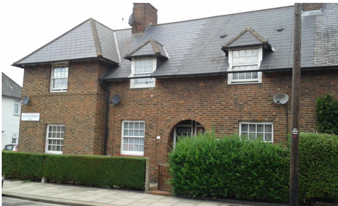
Gutters run in front of the first floor hipped dormer windows in Osmund Street.
