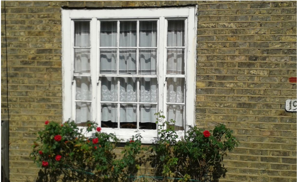
Original timber sash windows at No.19. The mullions are more slender than modern Upvc replacements.
