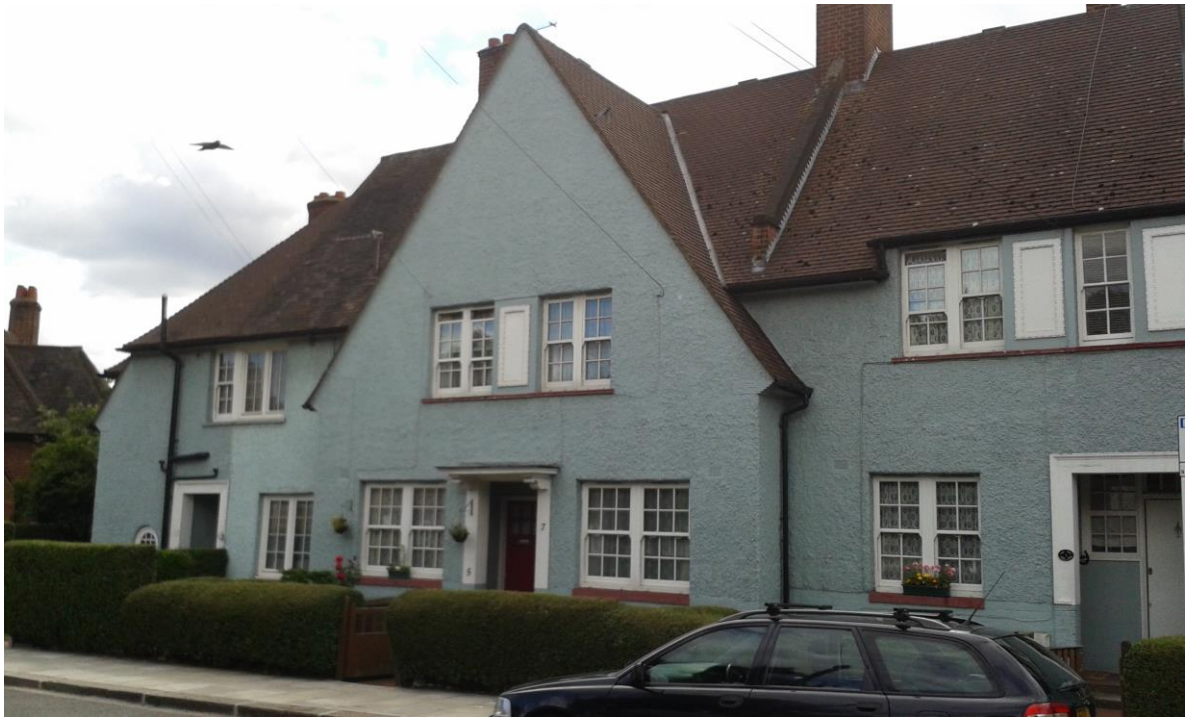
Original painted pebble dash nos.1-23 Fitzneal Street. Painted timber panels between first floor windows.
