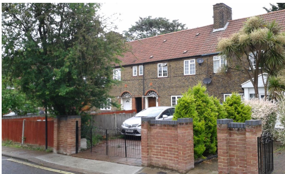
Distinctive multi-paned fanlights above entrances to houses in Primula Street, one fanlight is obscured by an inappropriate modern porch (right) and most of the garden of another is given over to car parking.
