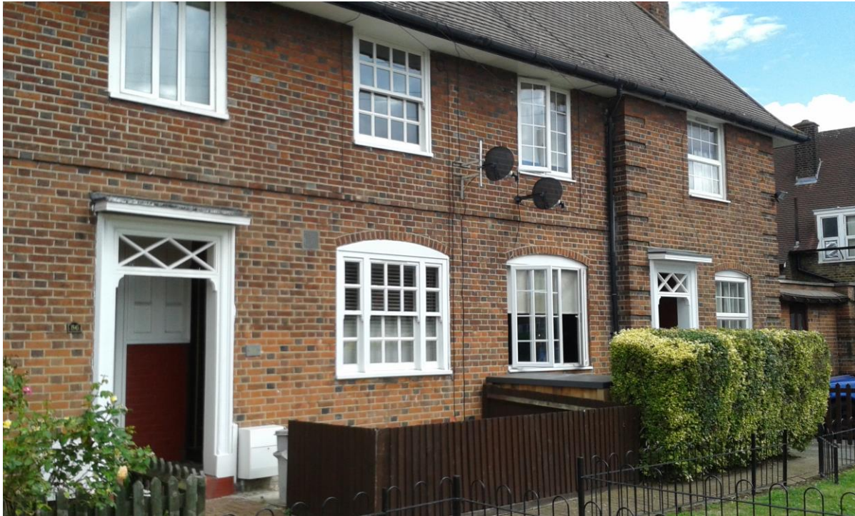
Distinctive arched window heads. Nos. 50-68 (even) Fitzneal Street. Full height bays have a brick relief detail. Some timber mullioned sash windows remain.
