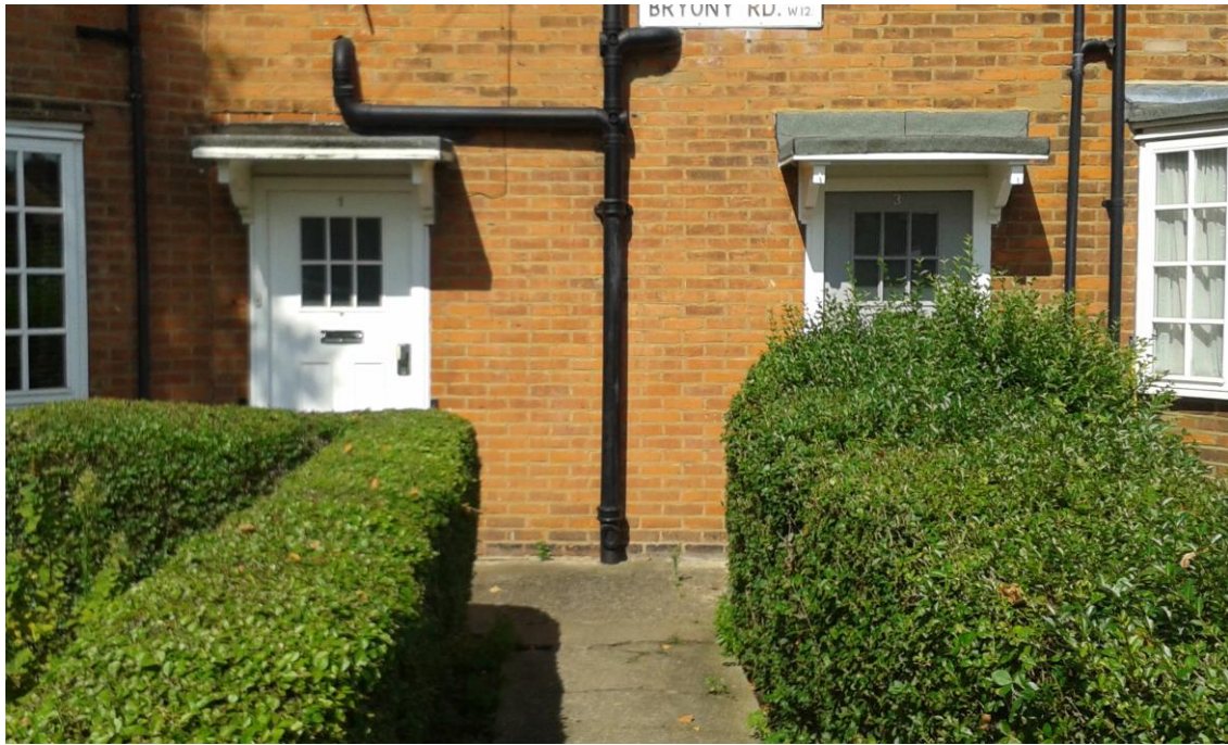
Timber panelled doors with a glazing panel subdivided by glazing bars are a characteristic of the conservation area, Nos. 1 and 3 Bryony Road.
