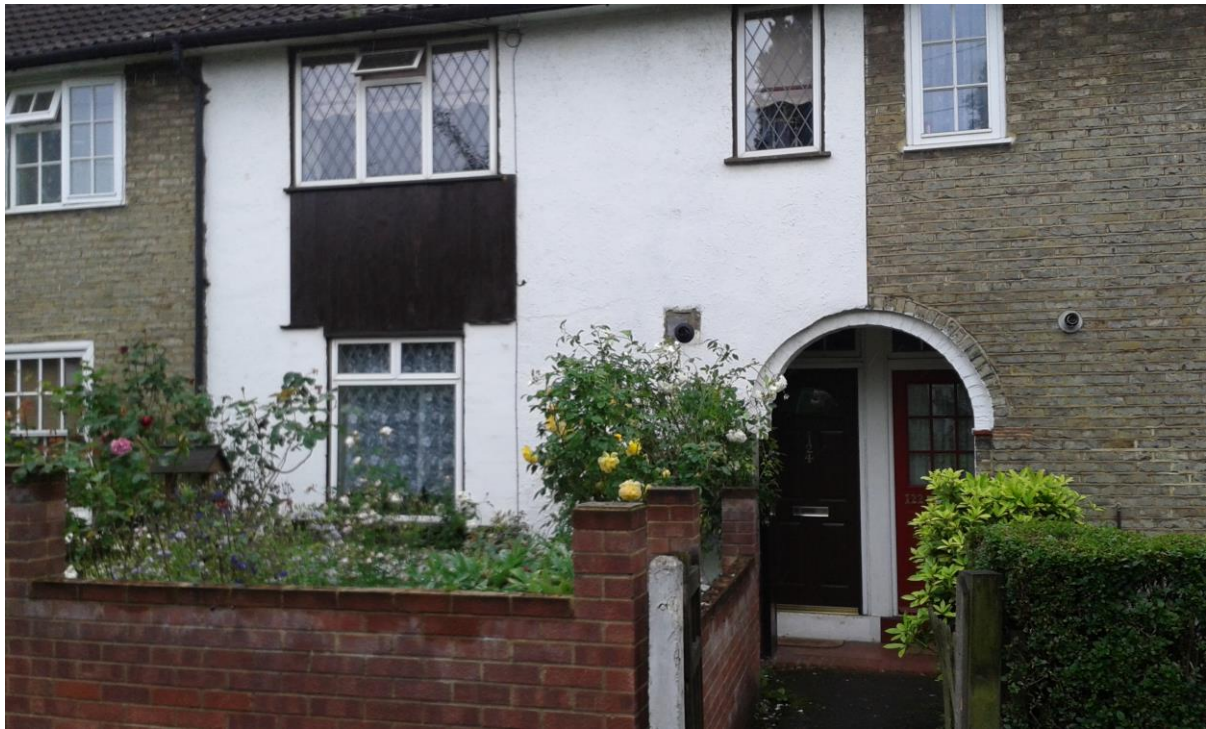
Inappropriate painted façade with leading light windows and timber cladding. Bentworth Road.
