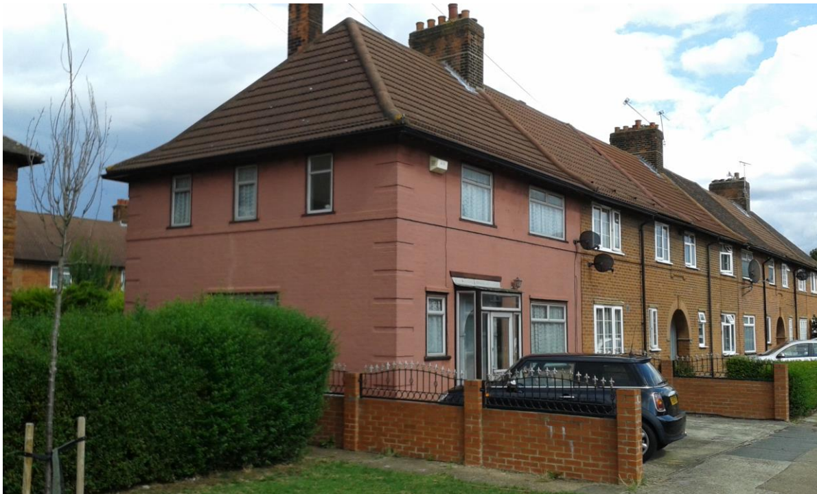
Painted facades on No.24 Daffodil Street together with a modern glazed porch and inappropriate replacement windows diminish the uniformity of the terrace. Fortunately, the string course and the brick work relief detail on the corner are still visible under the paint.
