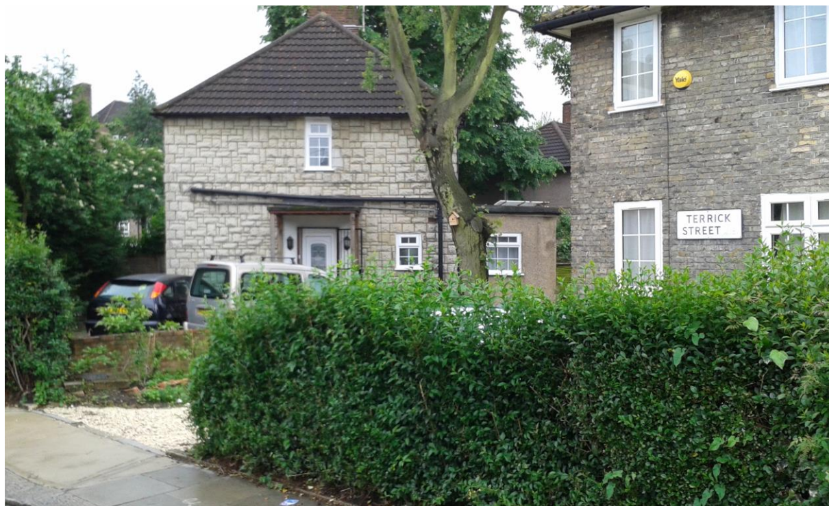
Inappropriate stone cladding on No.1 Terrick Street.
