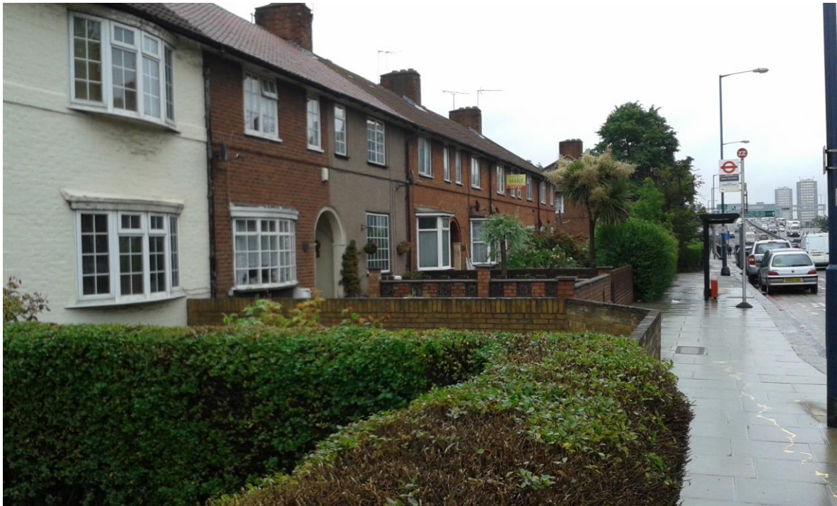
Long terraces laid out along the north side of Westway. Inappropriate insertion of curved window bays and a painted brick façade and a pebble dashed façade undermine the unity of the terrace.
