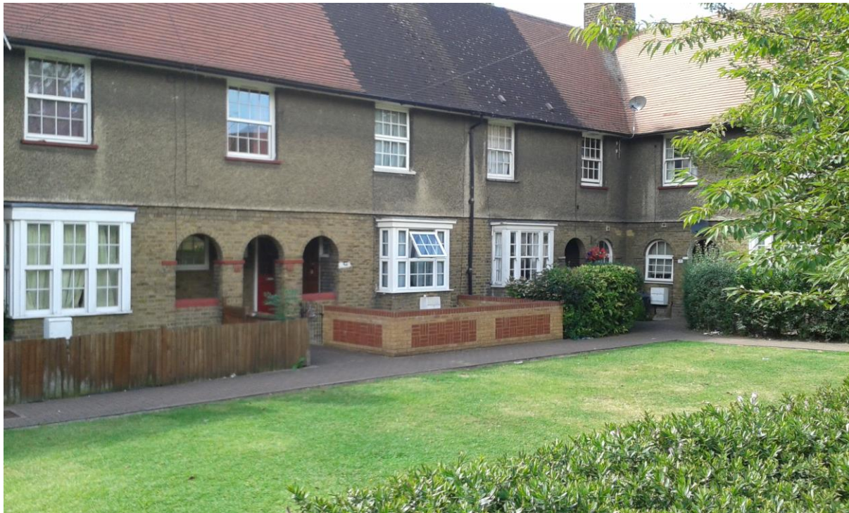
Nos. 79-119 Henchman Street, original pebble dash on first floor facades. Triple arched porches flanked by window bays.
